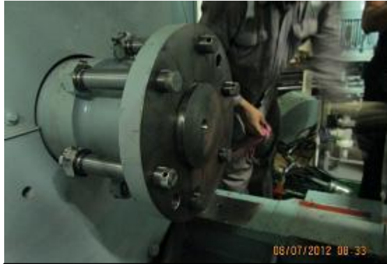
No need to remove whole reamer bolts
